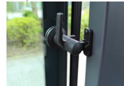
Side panels can be lifted out
